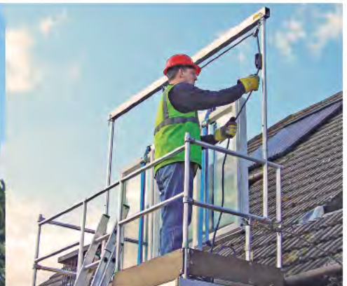
Hoisting to final position
