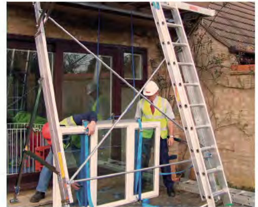
Attaching the new window
