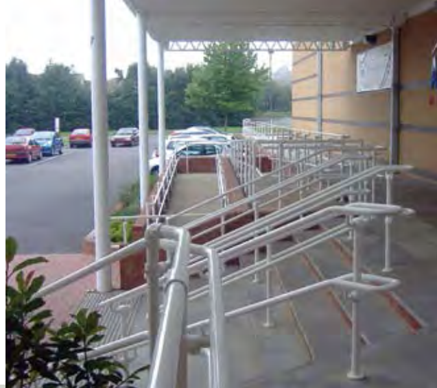
Right: ADA Compliant Railing for Public Access
